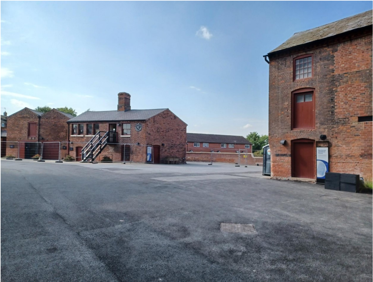
-View from West side of shop entrance looking at Dye House, to the right –
